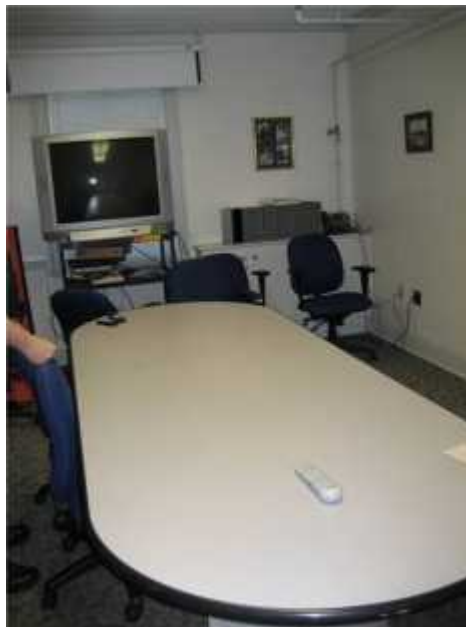
Photo 4. View of the EOC at the Blount House. The room is too small to house a fully staffed EOC and has several unreinforced windows.
