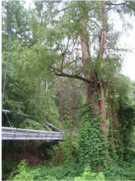
Photo 3. View of large trees overhanging the Greenville Run utility crossing. These trees should be removed as this utility corridor is essential in supplying the main campus with power and heat.
