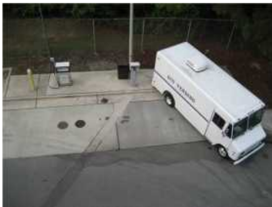
Photo 5. View of fuel pumps exposed to vehicle impacts.
