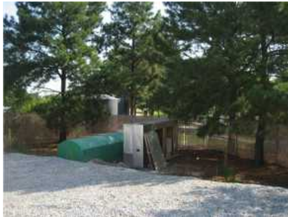
Photo 5. View of trees surrounding the well pumps.
