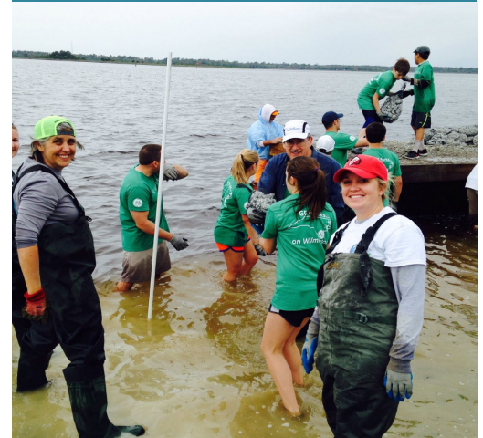
Masters of Coastal & Ocean Policy (MCOP) students constructed an oyster sill to dissipate wave energy at Carolina Beach State Park as part of their service learning assignment for N.C. Coastal Issues & Experiences course.
