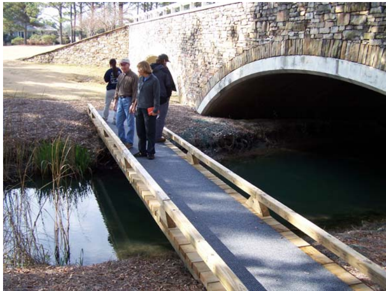
Plate 5. Course outflow site from small bridge, EP-BROUT.
