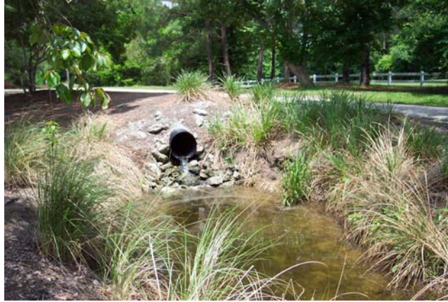
Plate 1. Course input site EP-PNRIN; Porters Neck Road beyond white fence in background.
