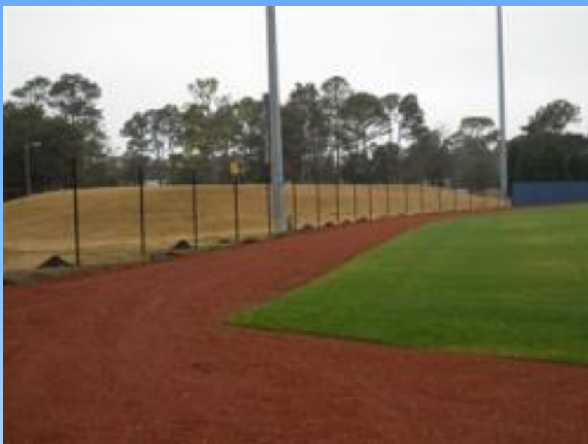
Removal of outfield fence.
