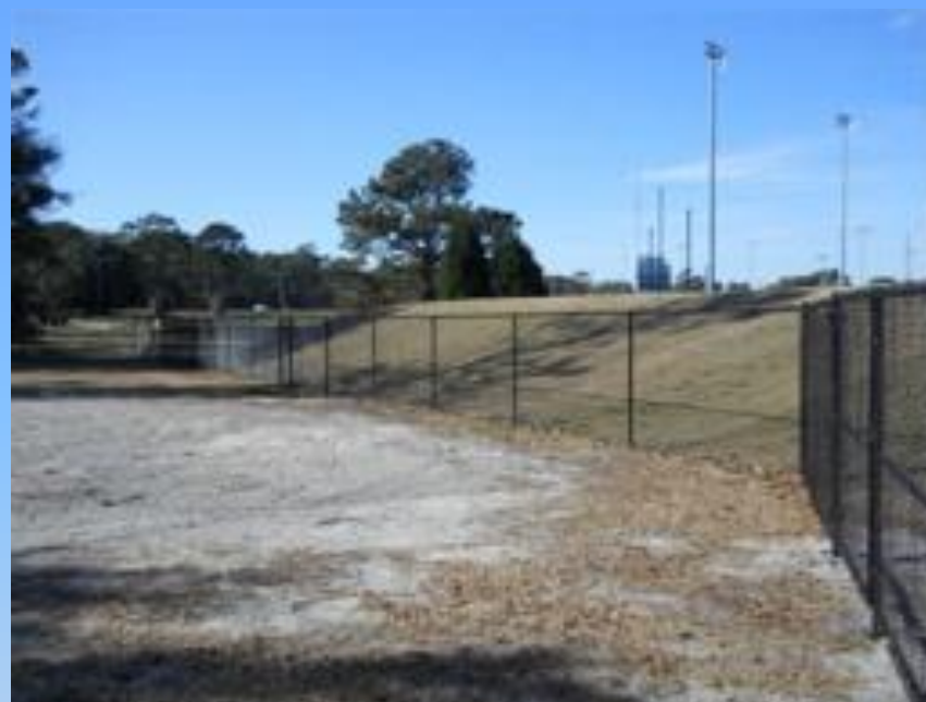
New security fence surrounding the outfield berm.
