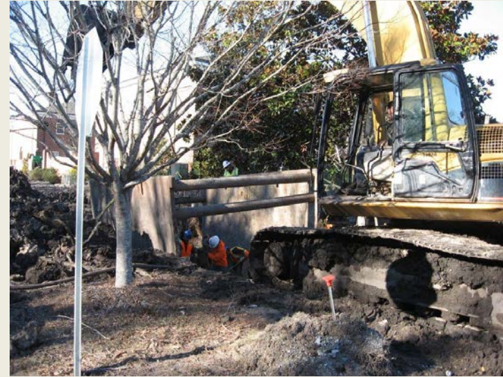
Connecting the HW & CW Piping to the Plant
